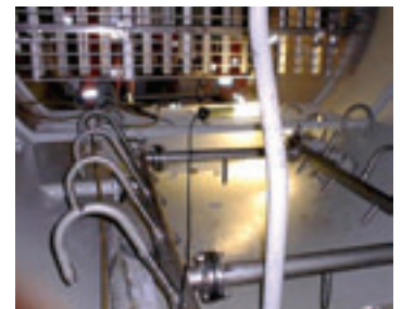
Installation of Sandwash System
