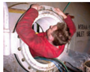
The BA Inlet Separator Vessel and its only Manway Access
