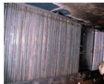
Installation of ZP-210 "V-bank" Vane Pack
